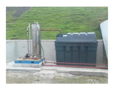
VGS - The Vertical Gravity Separator is a compact, cost effective unit developed to separate non-emulsified oil and water
